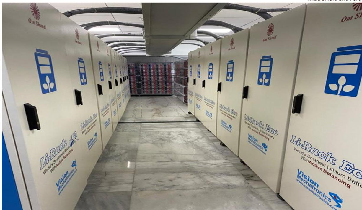
Figure 4: Mega Watt Scale Hybrid Energy Storage With Lithium-Ion Battery
